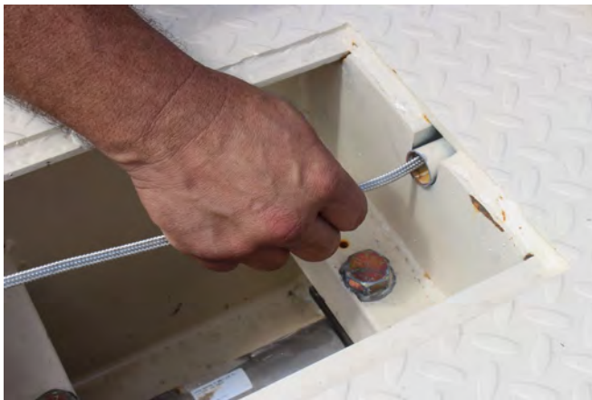
Insert the load cell cable into the scale conduit.
